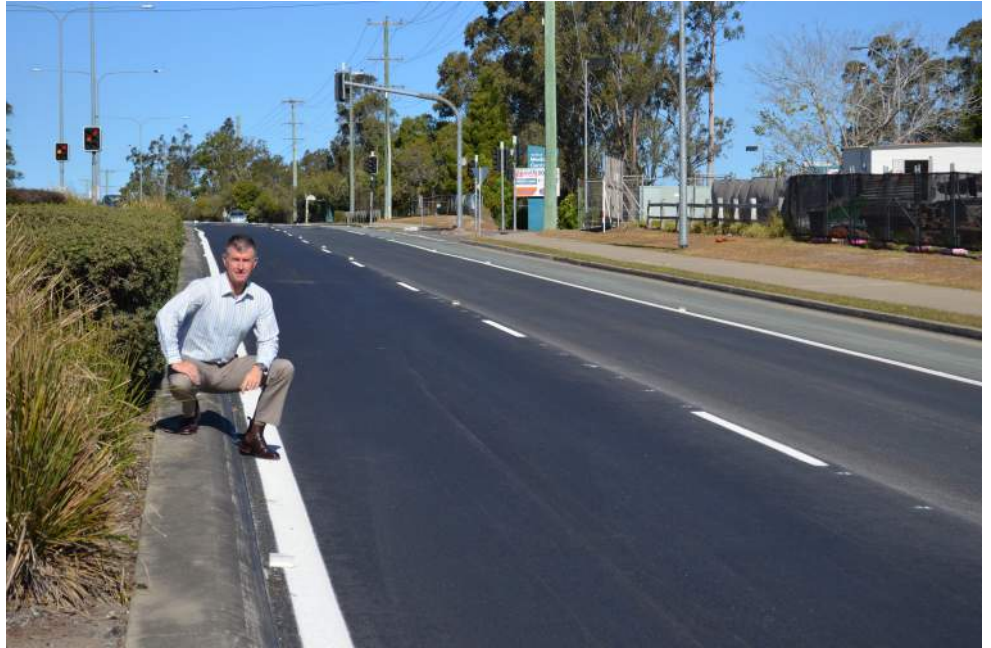
Inspecting the newly resurfaced Old Northern Road, Albany Creek
